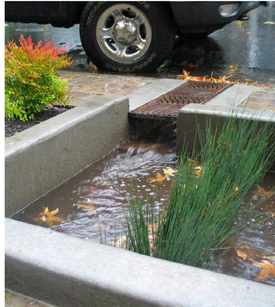
*Stormwater planters filter runoff into the ground water, keeping it from being funneled into storm sewers, lakes, and streams.*
