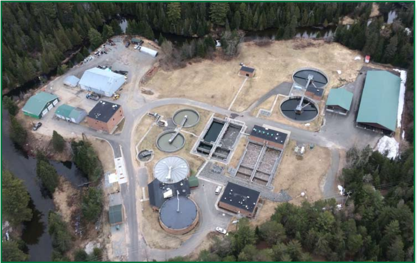
Aerial view of the Village of Lake Placid Wastewater Treatment Plant. Photo: Adirondack Council Staff
