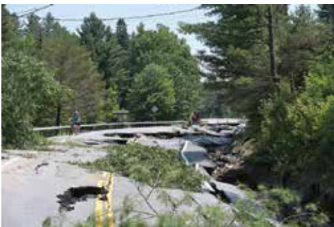
Road damage after severe flooding in Long Lake PHOTO: DEPT. OF ENVIRONMENTAL CONSERVATION
