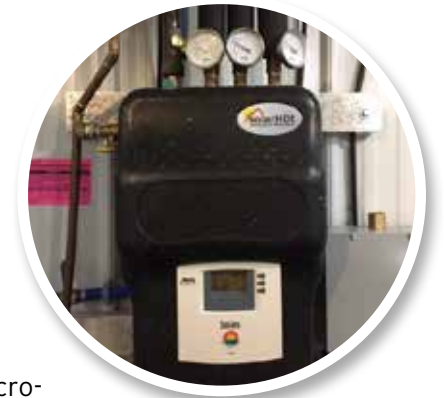
Solar hot water control panel
