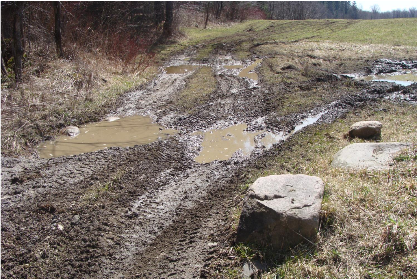
Damage to Whetstone Gulf State Park
