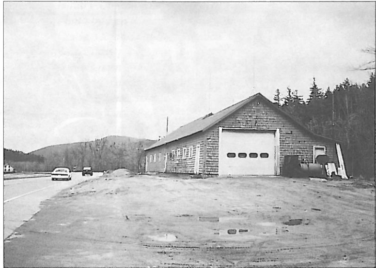
The Keene Town Highway Department garage on Route 73 lies right next to a stretch of the Ausable River about to be turned over to the state for addition to the Forest Preserve. It will be removed, thanks to a federal grant obtained by the APA. Photo by John Sheehan.
