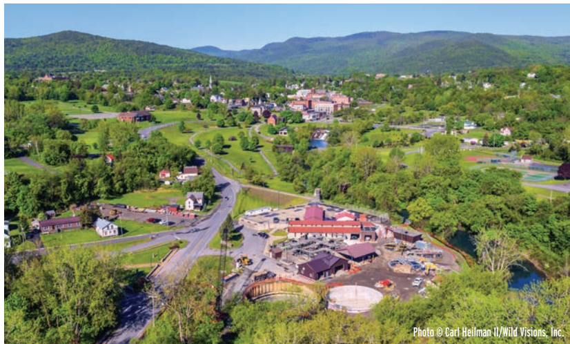
Ticonderoga Wastewater Treatment Plant along the La Chute River
