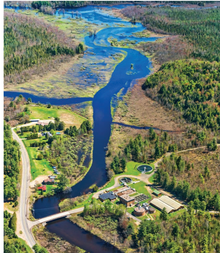
Saranac Lake Wastewater Treatment Plant
