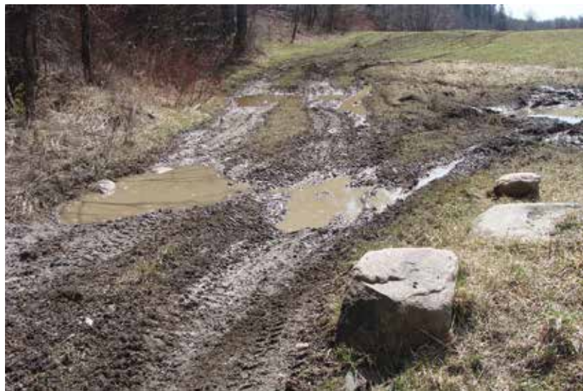
— One day worth of ATV damage at the Whetstone Gulf State Park on the western edge of the Adirondack Park
